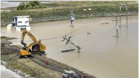
Unison crews work to get power back to Napier on Friday.
