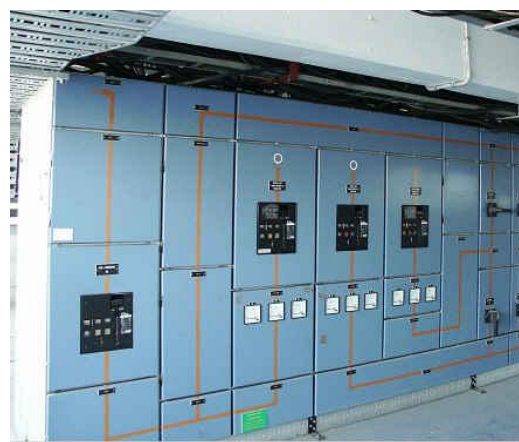
Main 415 V LVAC switchboard
