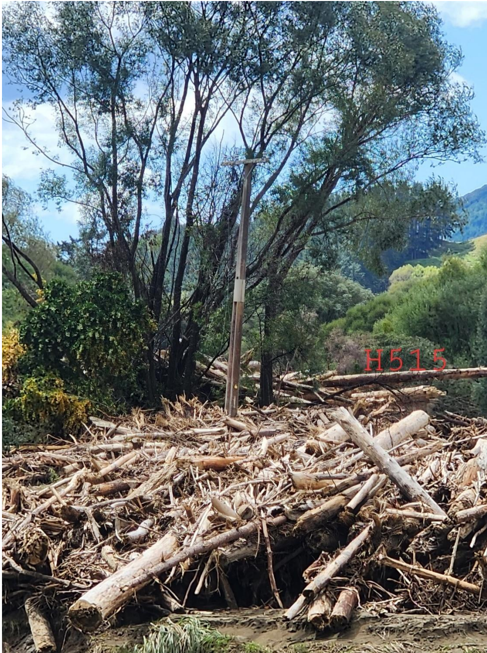
Ihungia road- tree through lines after flooding and slips
