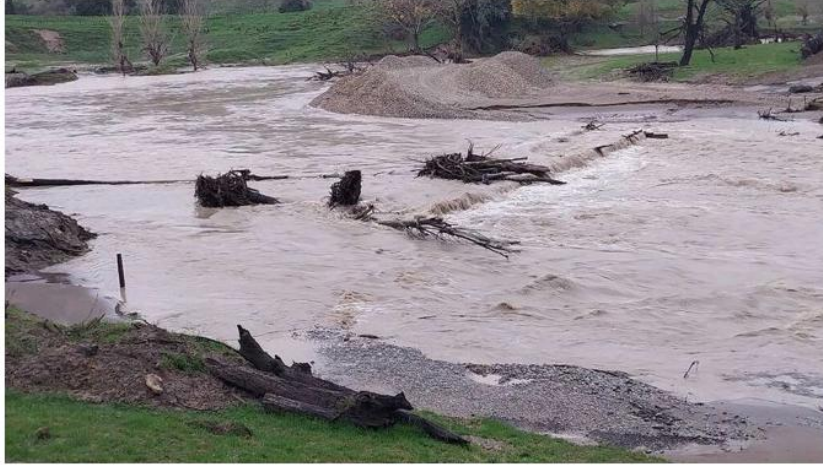
The temporary bridge on Bushy Knoll Rd, Tairāwhiti, is impassable - but hanging on - after heavy rain. Photo / Supplied
