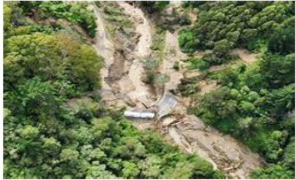
Photograph 7: Roading impacted in Tairāwhiti
