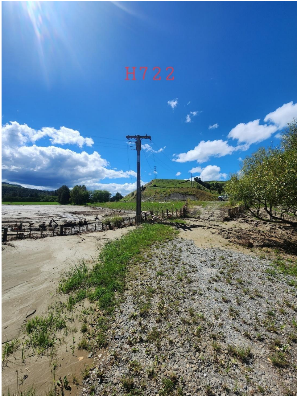
Waiapu Road- flooding and slips
