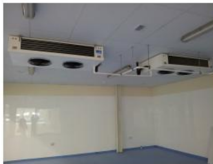
Refspecs evaporator in Fish Prep coolroom
