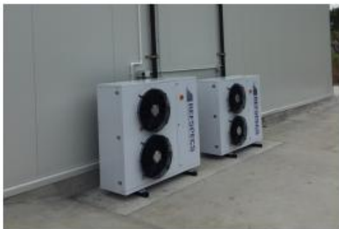
Typical installation of pre-assembled units for milk depot storage
