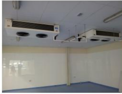
Refspecs evaporator in Fish Prep coolroom
