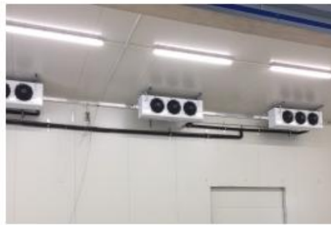
Typical installation of pre-assembled units for milk depot storage
