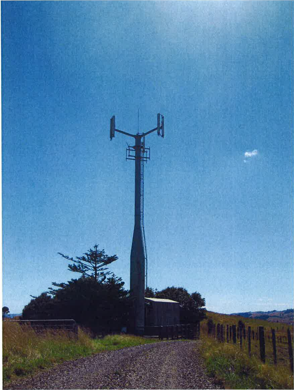
VNZ Clevedon 2G only and either go in between existing antenna or swap to x-pol's and use spare mount.
