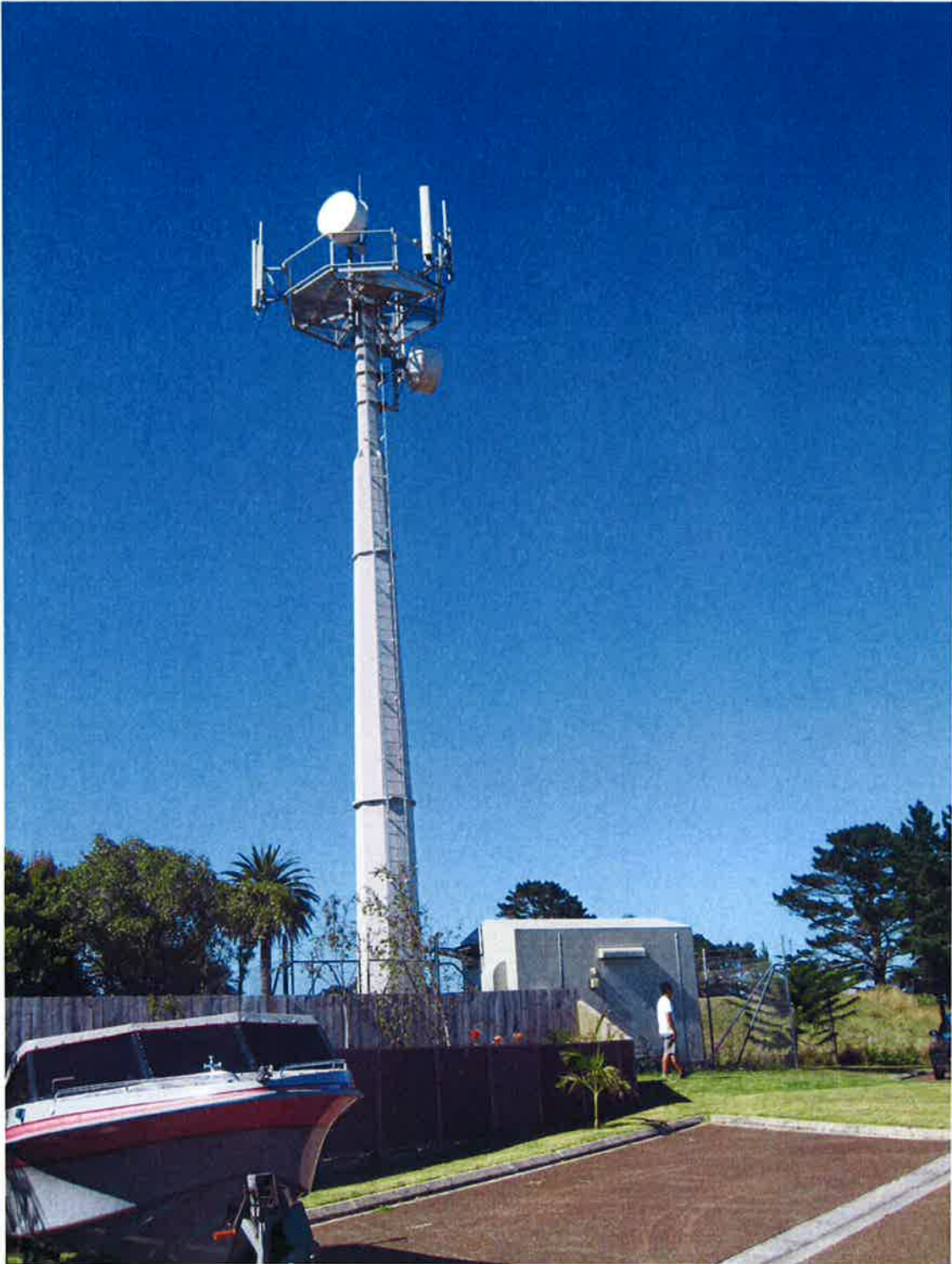
VNZ Beachlands Good example of 2G with 3G overlaid on top (2G larger x-pol antenna on right, 3G smaller x-pol on left). Shows VNZ can use antenna minimization
